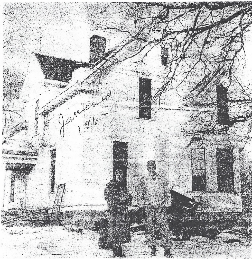
FIRE LAST THURSDAY EVENING destroyed the interior of this house owned and occupied by Mr. and Mrs. Bert Lee southwest of Fertile. The Lees stand in front of their house in which they and their seven children lost all of their possessions except the clothing they were wearing when they escaped from the burning house.
